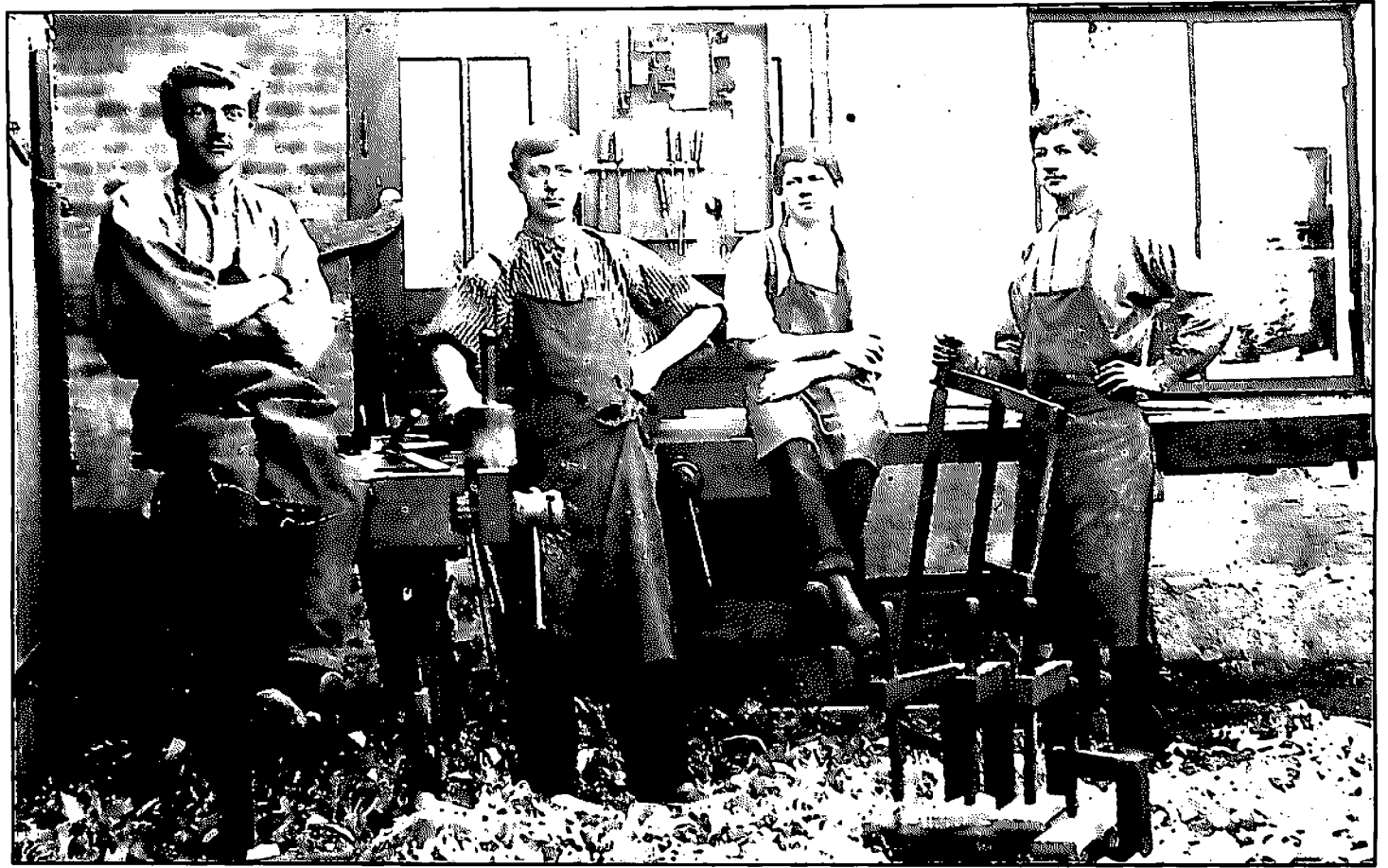
Victorian carpenters taking a break
